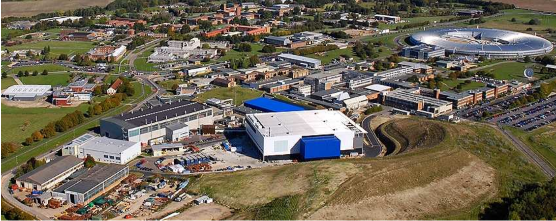
Figure 13.10: The Rutherford-Appleton Lab in Oxfordshire, UK. On the right, the large circular building is the DIAMOND synchrotron light source. The building on the left is the ISIS spallation neutron facility. This was the world's brightest neutron source on earth until August 2007 when it was surpassed by one in Oak Ridge, US. The next generation source is being built in Sweden and is expected to start operating in 2019. The price tag for construction of this device is over 10^9 euros.
