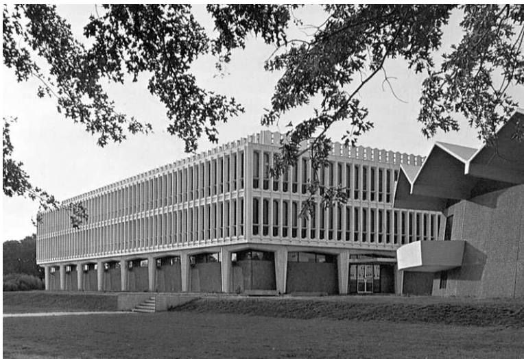
Figure 34 New Physics Building on Busch Campus
